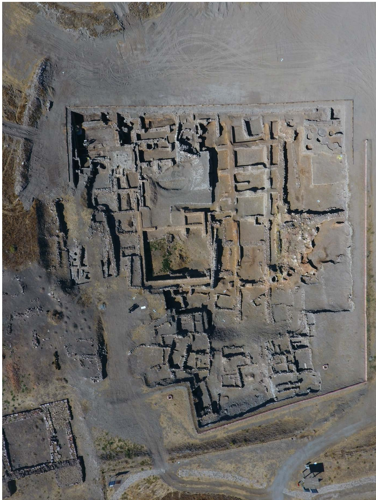
Fig.1 The building complex of Level XIII
